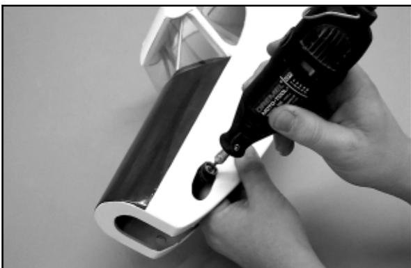
pair of pliers transfer the marks to the outside of the fuselage. Grip the pin tightly with the pliers, align the pin with the marks on the inside of the engine compartment and push it through the fuselage side and covering. This now shows you where to begin the holes. Use a Dremel® Tool and grinding bit to begin opening the muffler exit hole, a little at a time. Re-install the engine periodically to check the proper alignment of your work.
